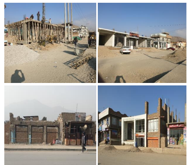
Figure 2: Still, the houses and shops of displaced families are uncompleted.
