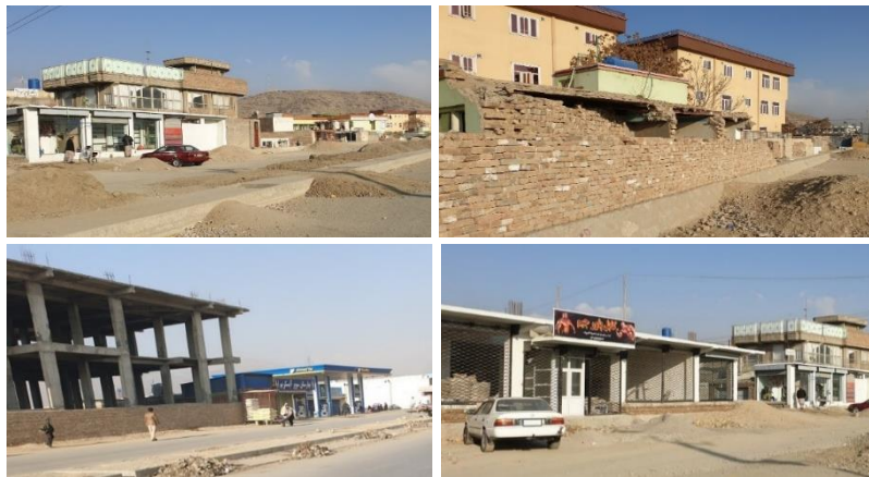
Figure 3: Many houses and shops are still under construction after displacement.
